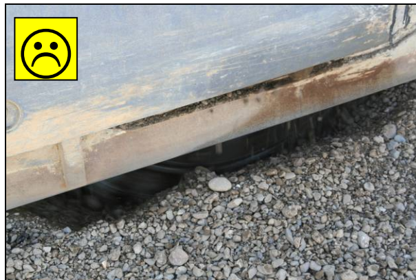
Figure 6.32: Material segregation during idling.
