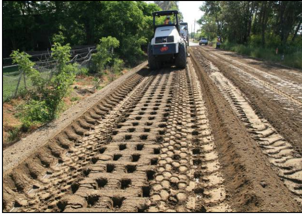
Figure 6.37: First padfoot roller pass impressions.
