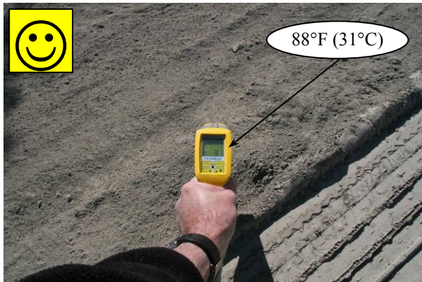
Figure 6.22: Portland cement temperature prior to recycling (warm).
