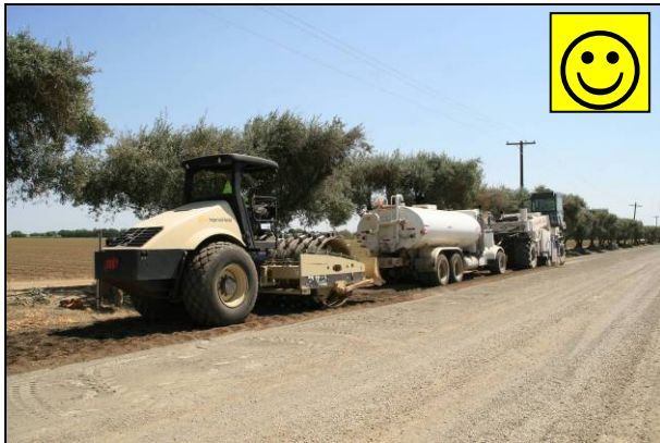
Figure 6.39: Desirable initial compaction procedure.
