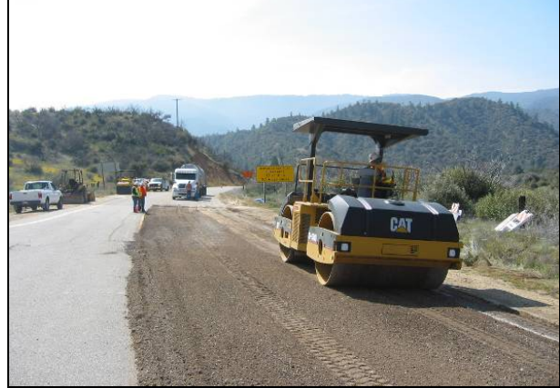
Figure 6.6: Smooth-drum roller.
