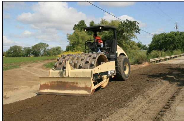
Figure 6.36: Using the blade to redistribute material in padfoot impressions.
