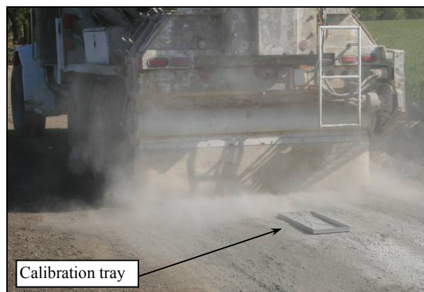
Figure 6.16: Checking active filler spread rate.
