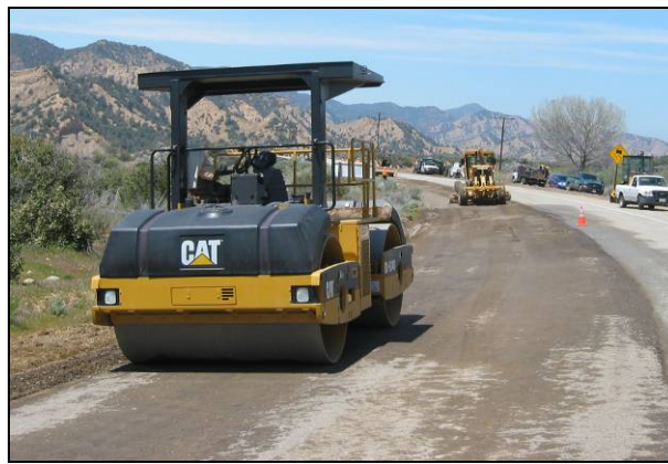
Figure 6.46: Smooth-drum roller behind grader.
