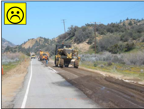
Figure 6.33: Water application between recycling train and roller before initial compaction.
