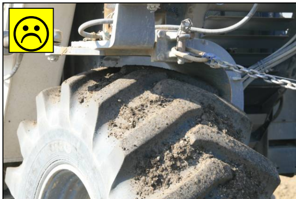
Figure 6.13: Unfoamed binder in recycled material.
