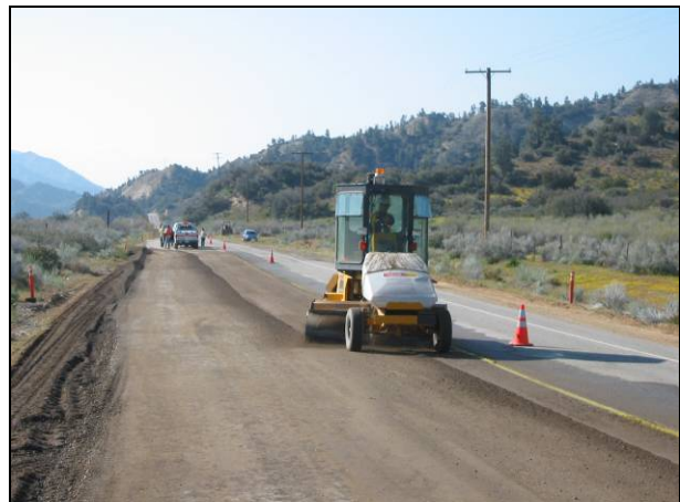
Figure 6.10: Mechanical broom.
